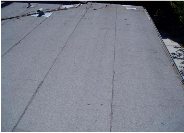
Rolled Roofing over the Rear Patio/Addition
