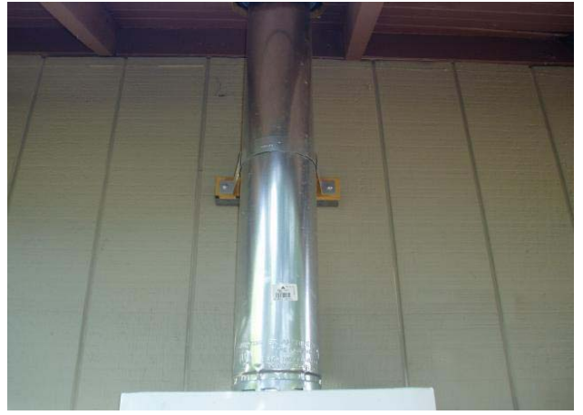
Tank less water heater connections (vent)
