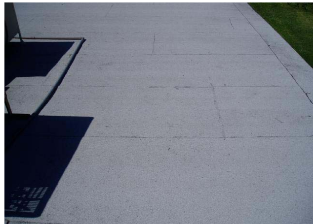
Rolled Roofing over the Rear Patio/Addition
