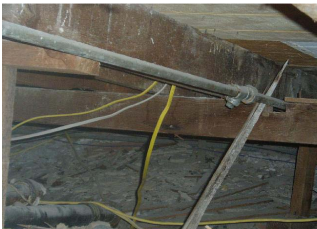
Need to support the gas and plumbing
