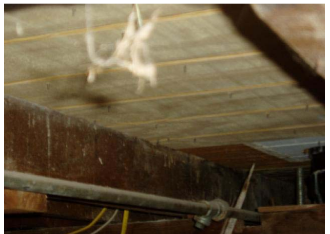
Need to support the gas and plumbing
