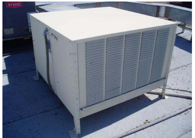
Rear addition Evap-Cooler (inop)
