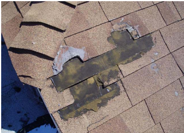
Patching observed on the rear portion of the roof line
