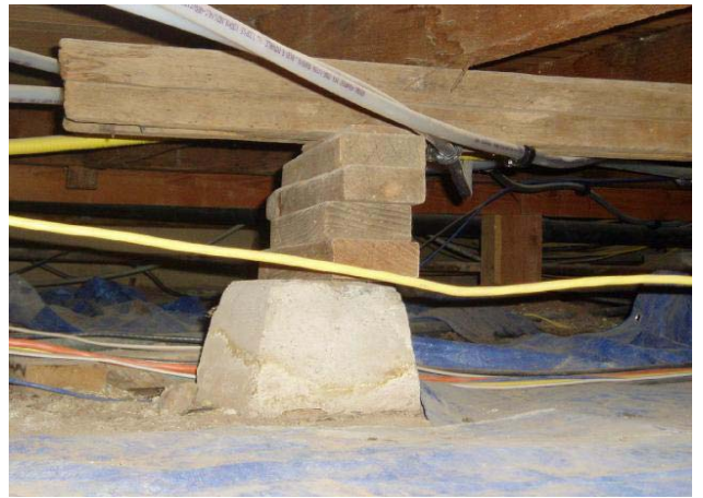
Need to adjust the supports
