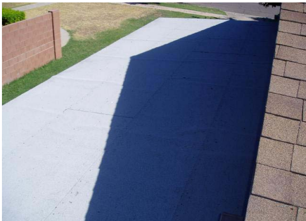
Rolled Roofing over the carport
