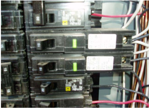
200 Amp. Electrical Main Breaker Panel (arch faults)
