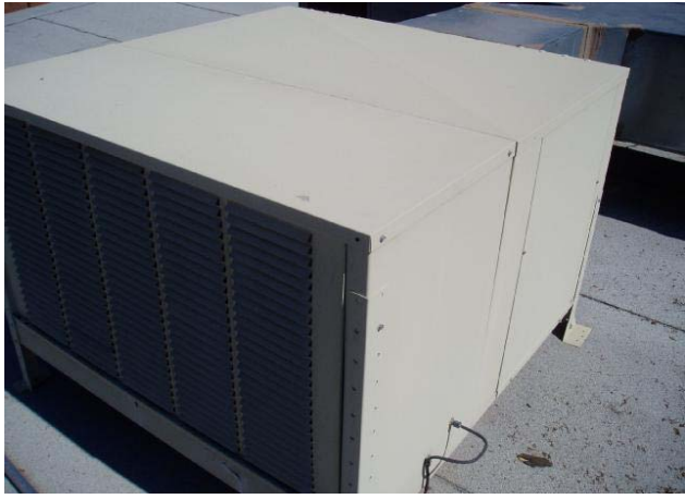
Rear addition Evap-Cooler (inop)
