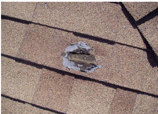
Patching on the rear roof line
