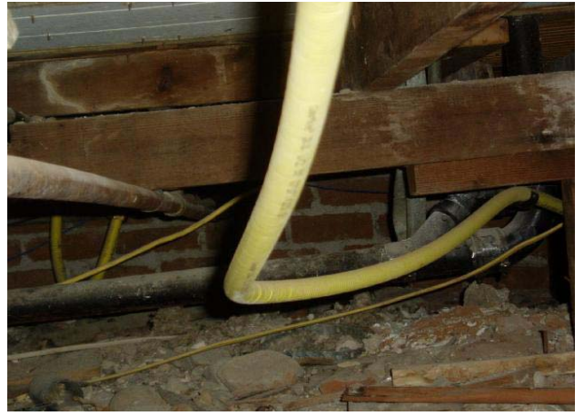
Need to support the gas and plumbing
