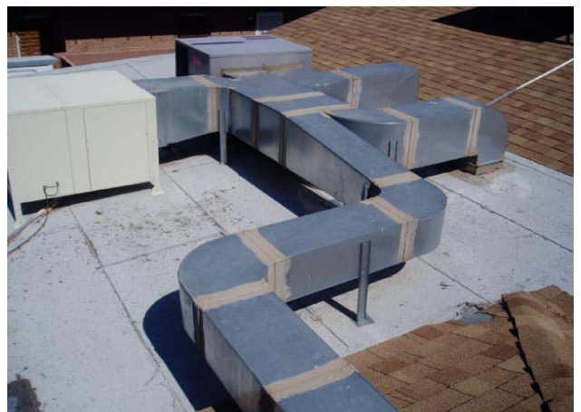
Duct systems over the rear addition
