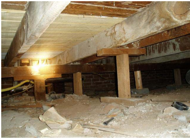
Adjust the floor supports
