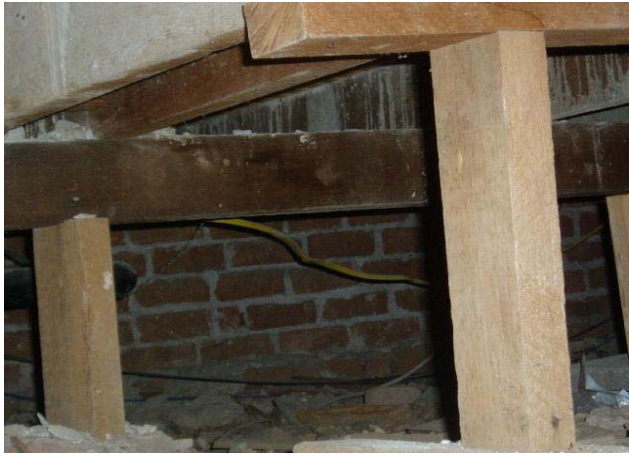
Adjust the floor supports
