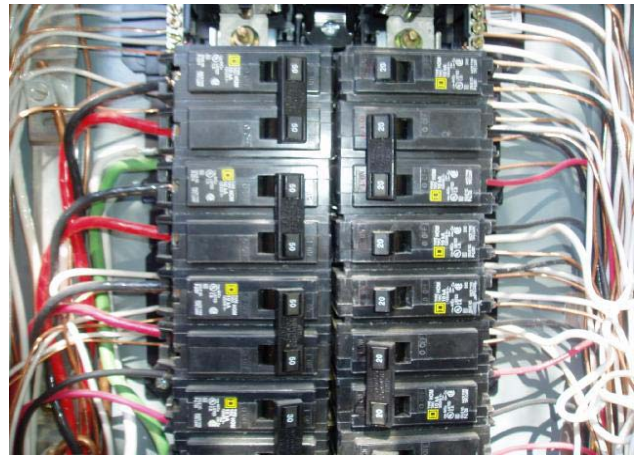
200 Amp. Electrical Main Breaker Panel
