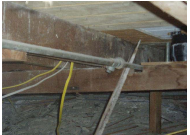
Need to support the gas and plumbing
