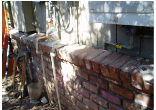
Loose brick and missing flashing
