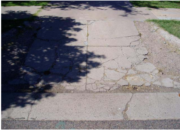
Deterioration on the front approach
