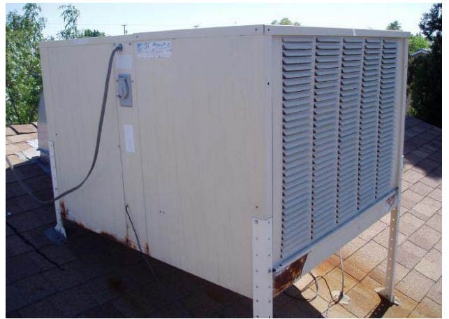
Evap-Cooler over the front portion of the home (inop)
