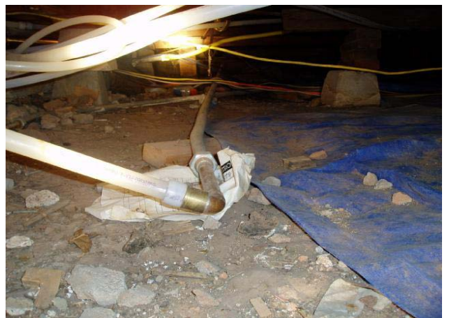
Need to support the plumbing
