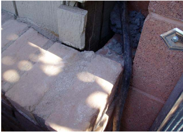
Loose brick and missing flashing
