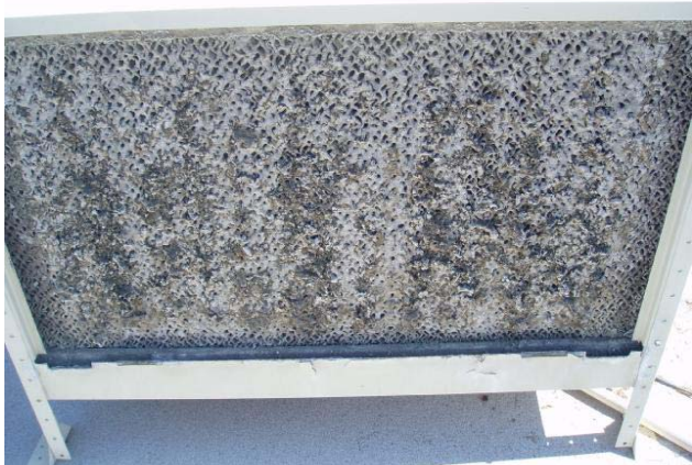
Rear addition Evap-Cooler (inop)
