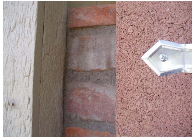
Brick siding and flashing
