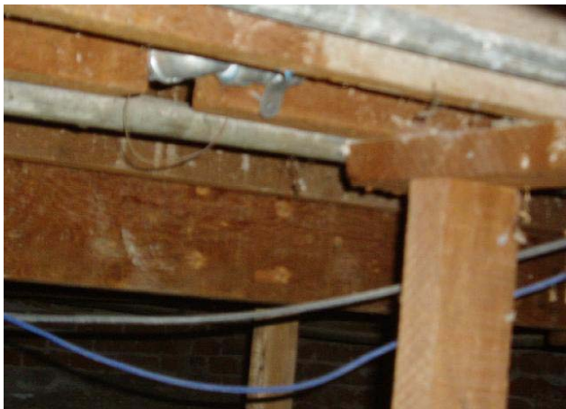
Supports for the flooring have been added
