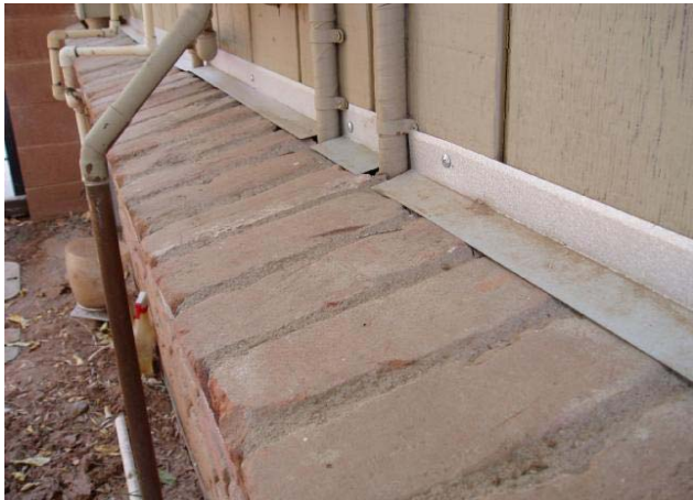
Brick siding and flashing
