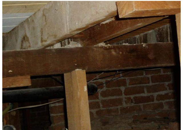
Supports for the flooring have been added
