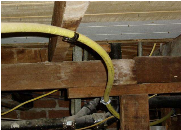
Supports for the flooring have been added
