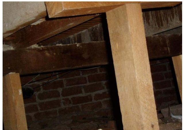
Supports for the flooring have been added
