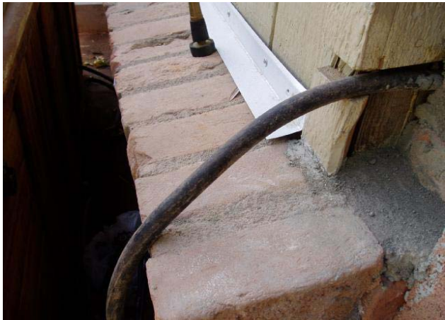
Brick siding and flashing
