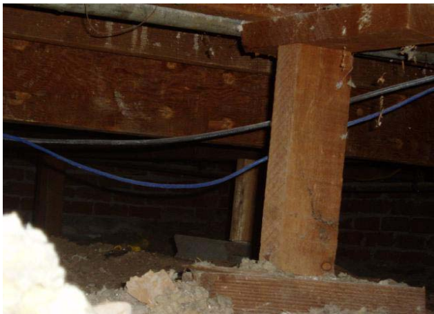
Supports for the flooring have been added
