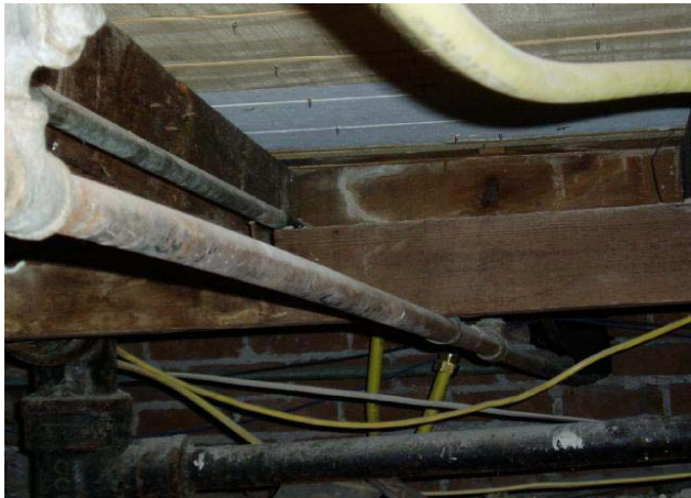
Supports for the flooring have been added
