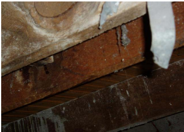
Supports for the flooring have been added
