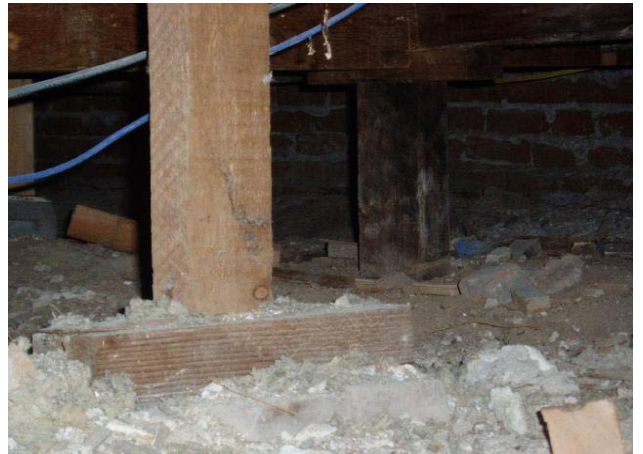
Supports for the flooring have been added
