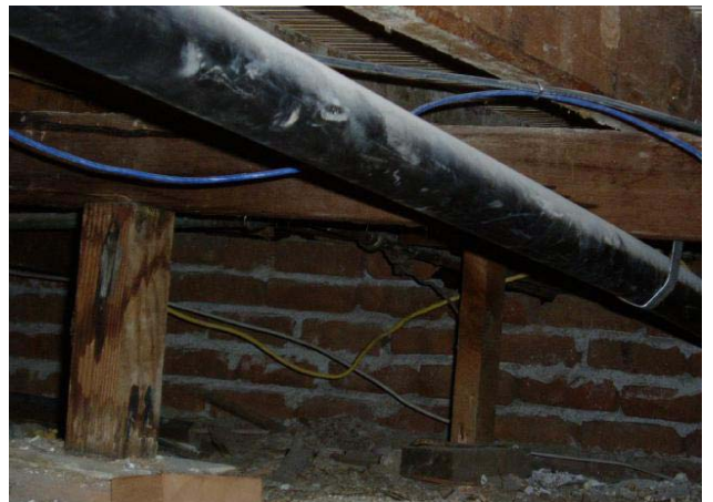
Supports for the flooring have been added
